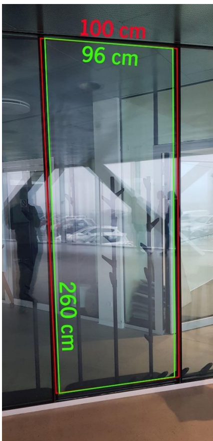
Picture 2 Location 1 (Main entrance closeup)
